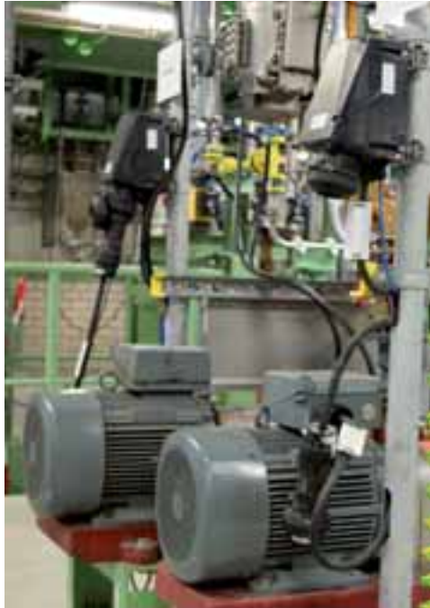
Electrical machines: Plug-in connection of pump drives, protection „nA“
