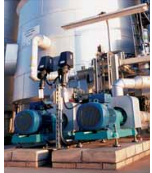
Light fitting for rod-shaped, bi-pin fluorescent lamps in the type of protection Ex-e for the illumination of a pump station. Three-phase Ex-e squirrel-cage motors as pump drives with plug-in connections (Ex-d/Ex-e).
