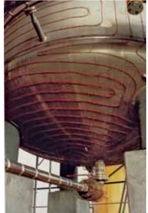
Example of a trace heating system
